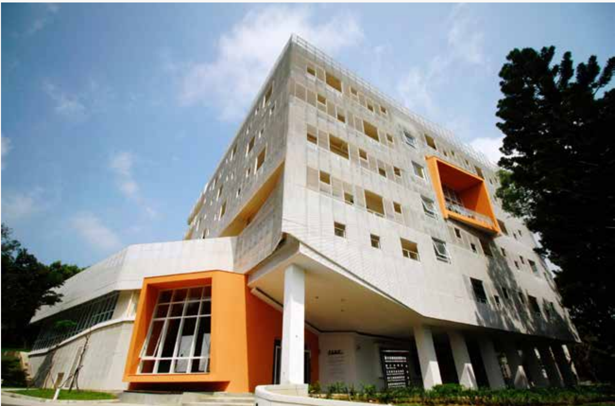
The Lee Tsen Min Building features an attractive white curtain wall which allows light and air in while blocking direct sunlight, thereby reducing air-conditioning costs by around 70 percent.
